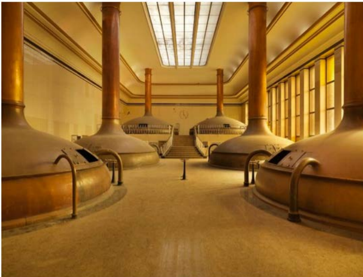
The Brew House, which will be opened to the public after refurbishment. Jens Ziehe, Berlin
